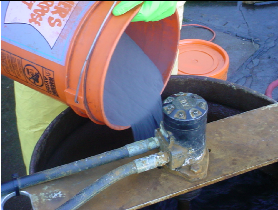
Photograph: 4 Adding powdered zero valent iron to water in a 55-gallon drum in preparation for injection (round one).
