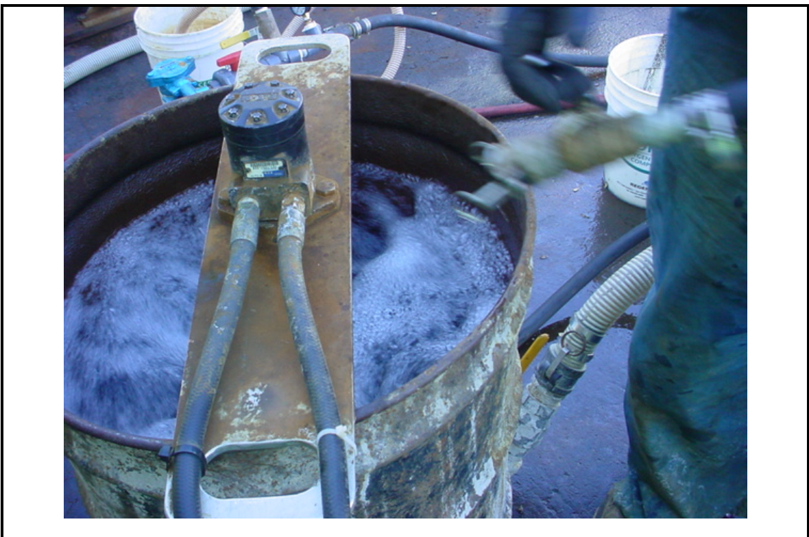
Photograph: 5 Vigorously mixing the zero valent iron with water to form a slurry prior to injection (round one). Spokane ANG5 ERM 242 nd CCSQ Spokane, WA
