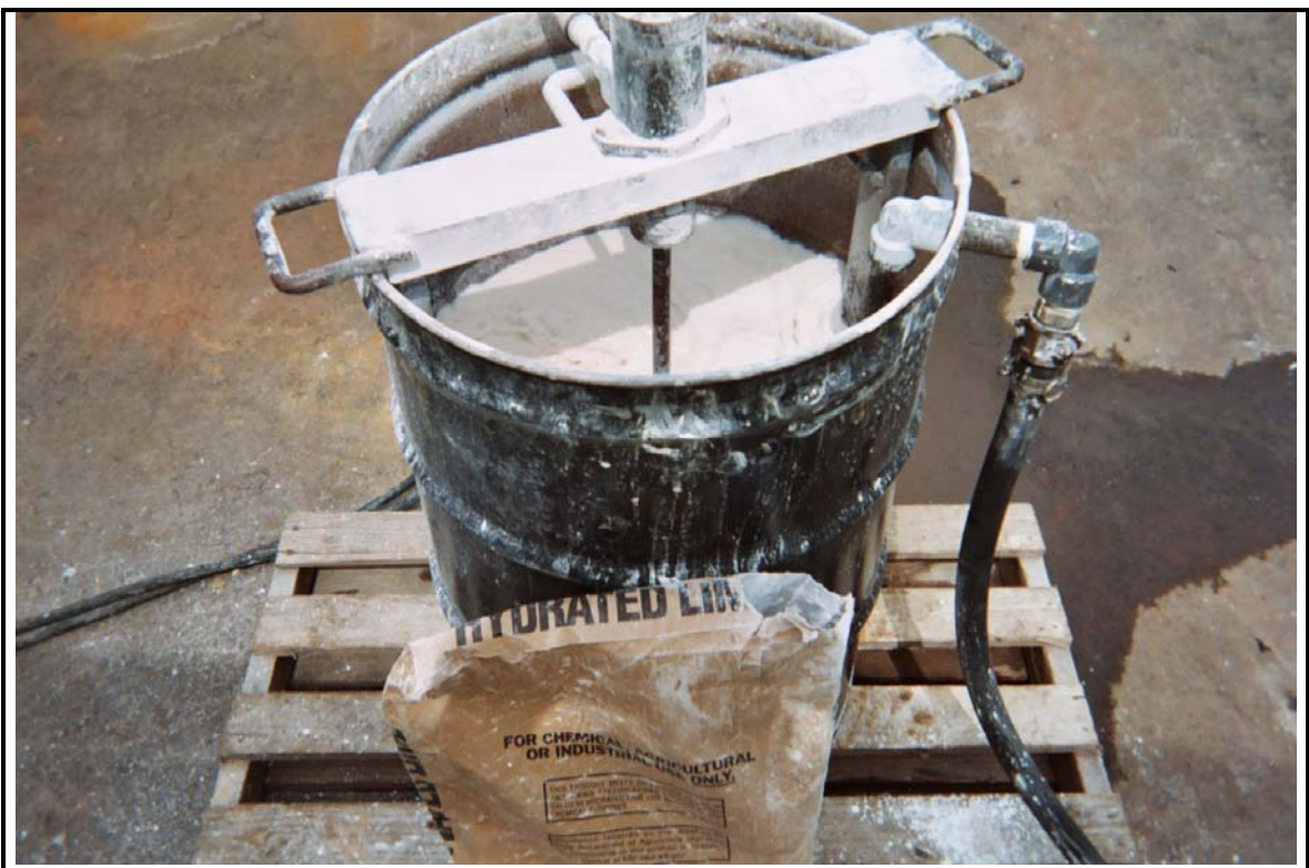
Photograph: 6 Adding powdered calcium hydroxide directly to sodium persulfate solution in a 55-gallon drum in preparation for injection (round two). Spokane ANG5 ERM 242 nd CCSQ Spokane, WA
